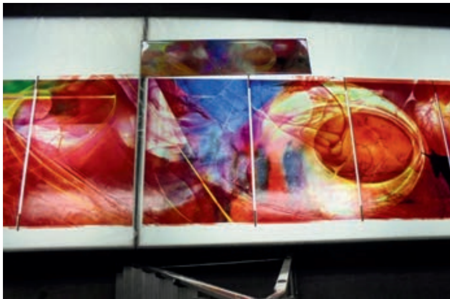
During construction of the Creation Window for Our Lady of the Angels Church in Scottsdale, AZ
